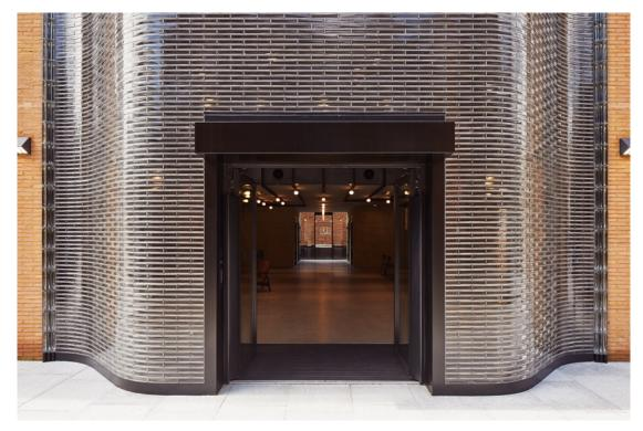
"The installation was incredibly accurate, gaining only a few millimetres of creep over the entire height. They were cast in low ion glass with a mottled texture, and about one third were hand polished on the long-side edge to offer vision panels and reflection points when the sun hits the glass brick feature wall," explains Pietro.
