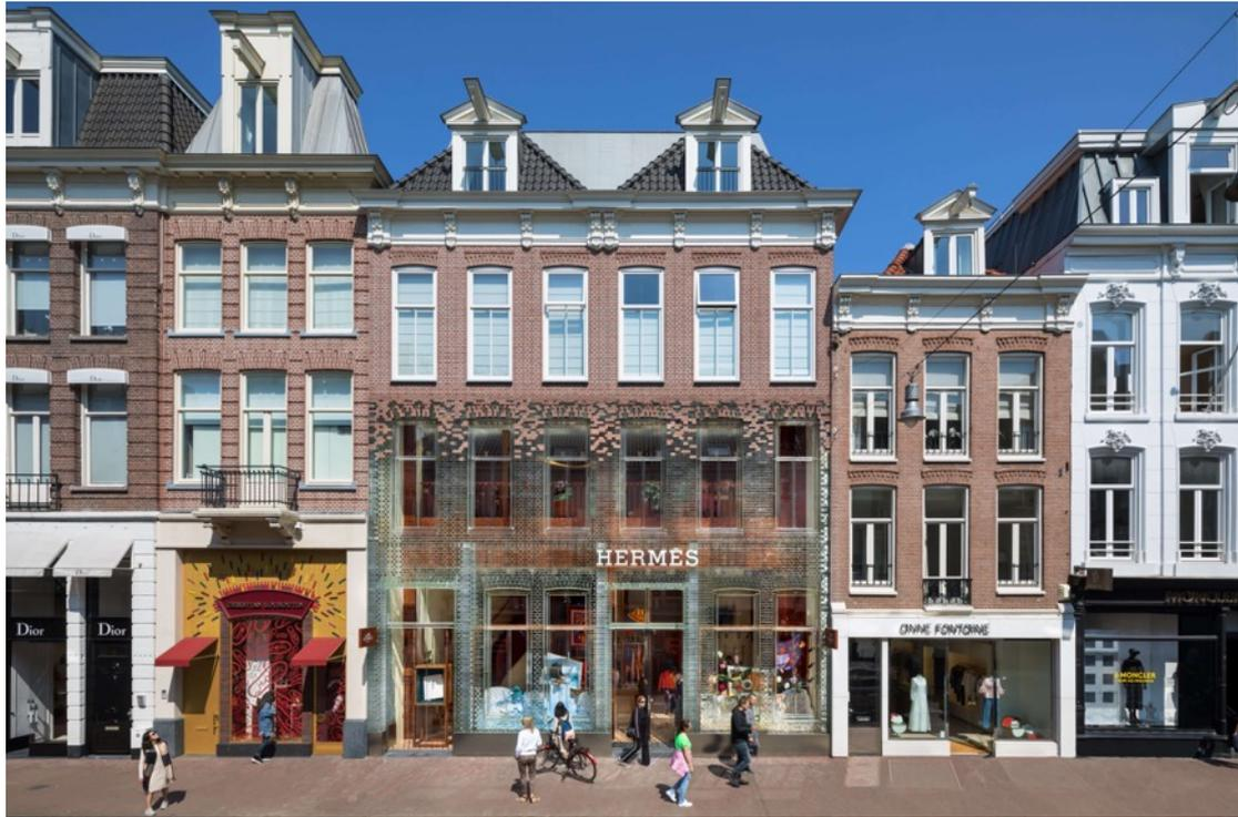
When Hermès moved in, some of the glass façade developed green tones, due to changes to the interior architecture (including construction of a dark tiled wall, and dark wood detailing) and the resultant reflectivity and light refraction from that, which has changed the façade appearance.
