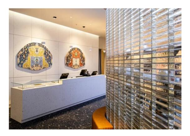
Made by Poesia Glass Studio, the unique curved wall includes smooth cast, clear, low iron glass bricks, made with a custom-mould and laid in a stack bond. A steel structure was built inside the glass bricks to hold up the long steel shelves that curve around the glass brickwork.
